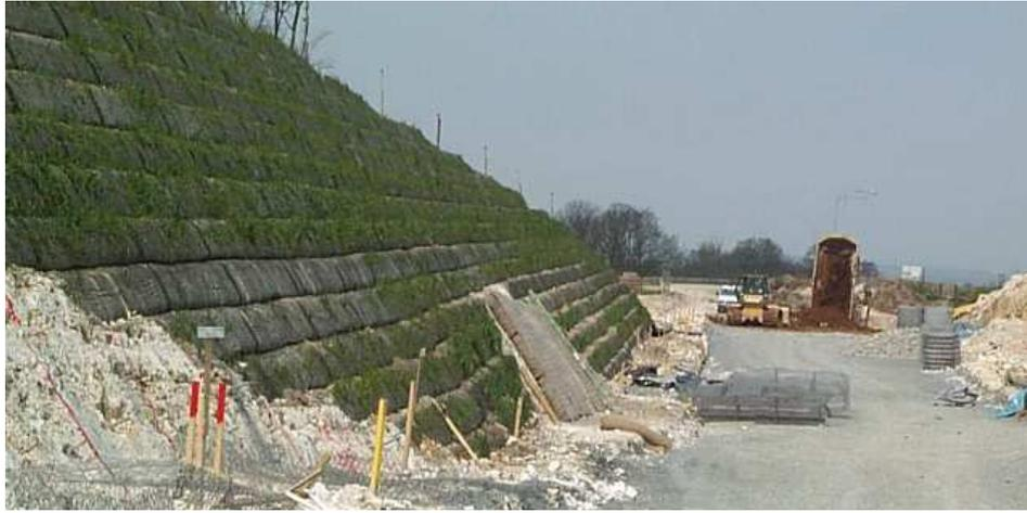
**Figure 7.** Steep slope with geogrid wrap-around facing
