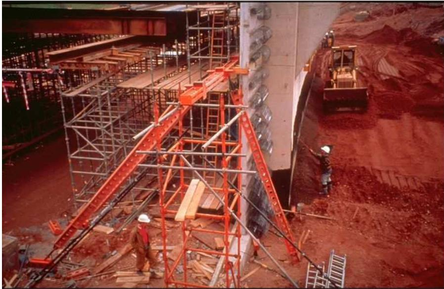
**Figure 2.** Full-height precast concrete facing
