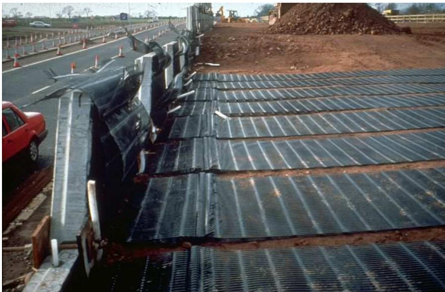
**Figure 1.** Vertical concrete facing with geogrid tails
