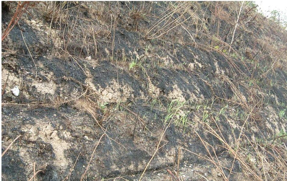
**Figure 8.** Steep slope with geogrid wrap-around facing- fire damage was easily repaired
