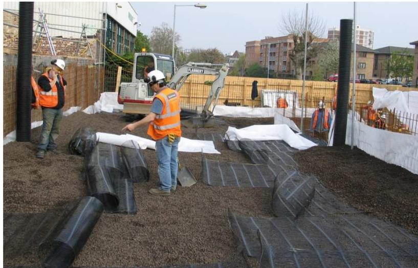
**Figure 10.** Geogrid-reinforced, very lightweight fill with steel mesh-face
