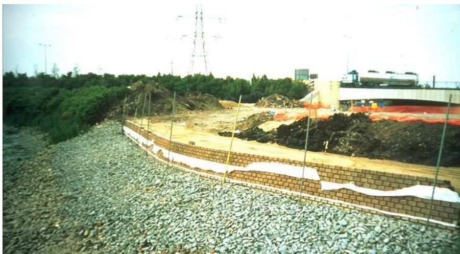
**Figure 4.** Geogrid-reinforced modular block-faced wall
