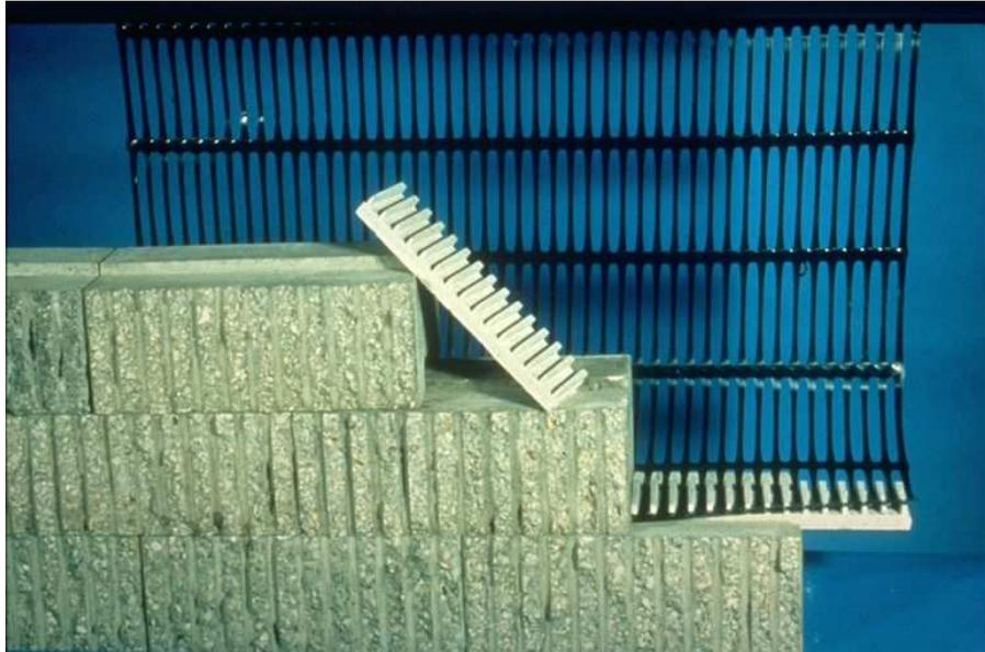
**Figure 5.** Modular block facing showing connection
