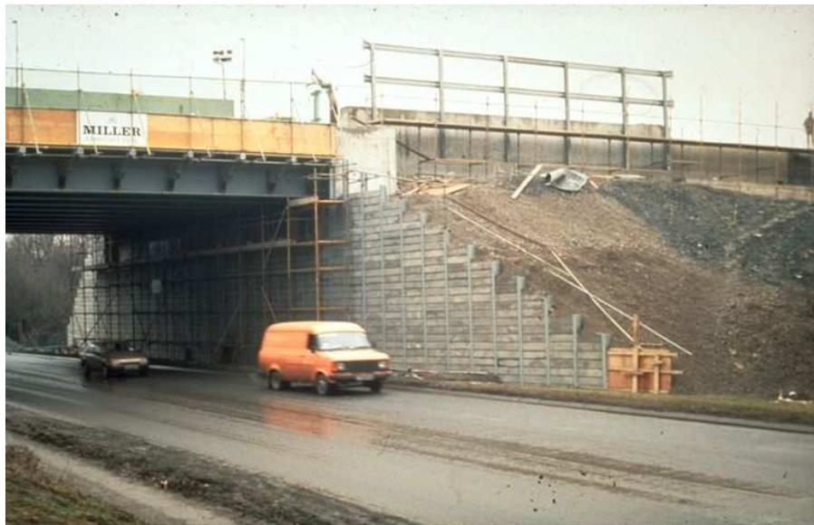
**Figure 3.** King post and plank-faced reinforced soil wall
