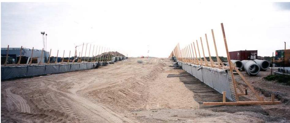
**Figure 9.** Geogrid-reinforced slope, mesh-faced at 78° to horizontal
