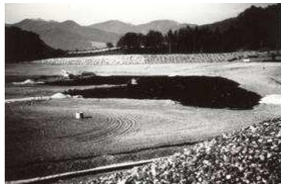
**Figure 7.** Three dimensional mattresses for foundation support system and used at a landfill in Hasham, Bavaria, Germany
