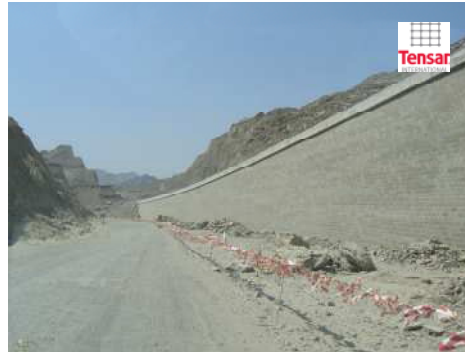
Figure 17. 20m high vertical wall
