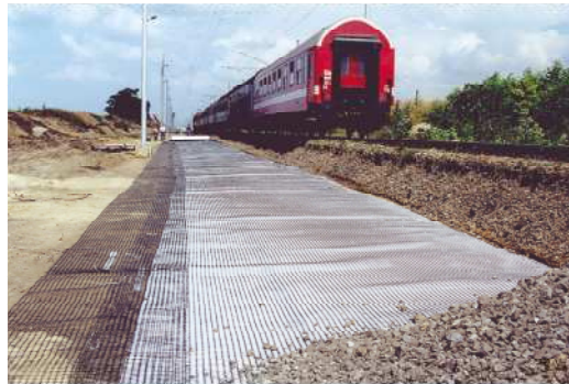
Figure 24. Railway ballast stabilisation
