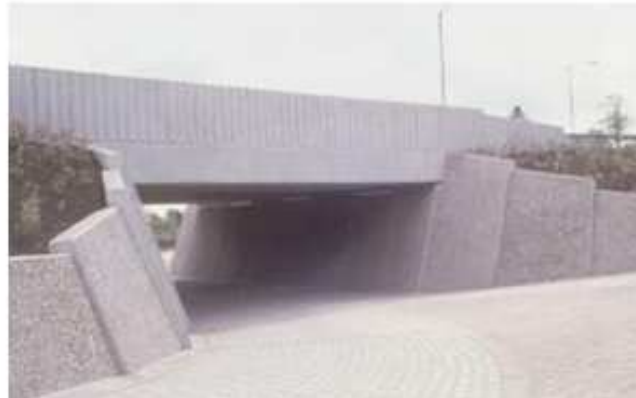
Figure 6. Stirling Bridge Abutments
