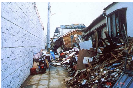
Figure 13. Unaffected geogrid reinforced soil structure
