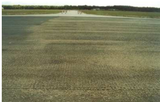
Figure 23. Airport runway resurfacing reinforcement
