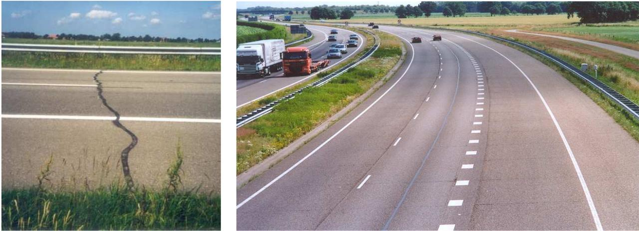
**Figure 2.** Typical reflective cracking on a cement treated base (left) and concrete slabs (right)
